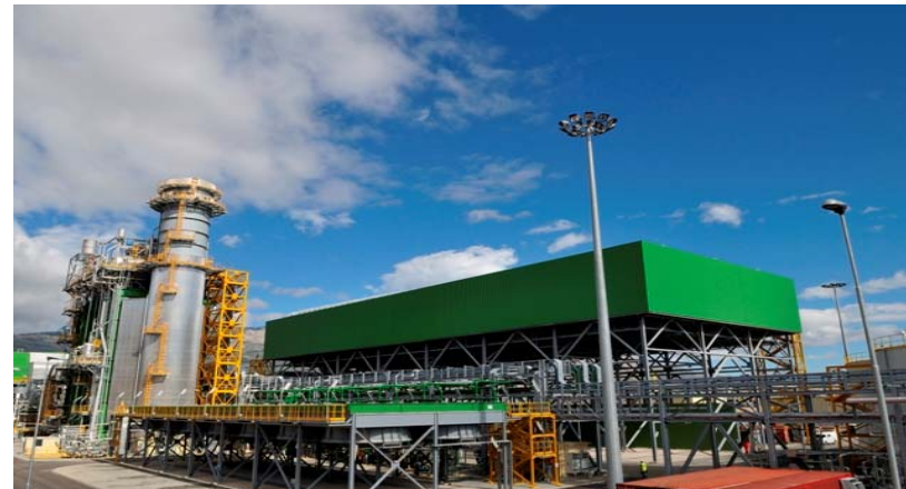
Thisvi 420MW CCGT power plant
