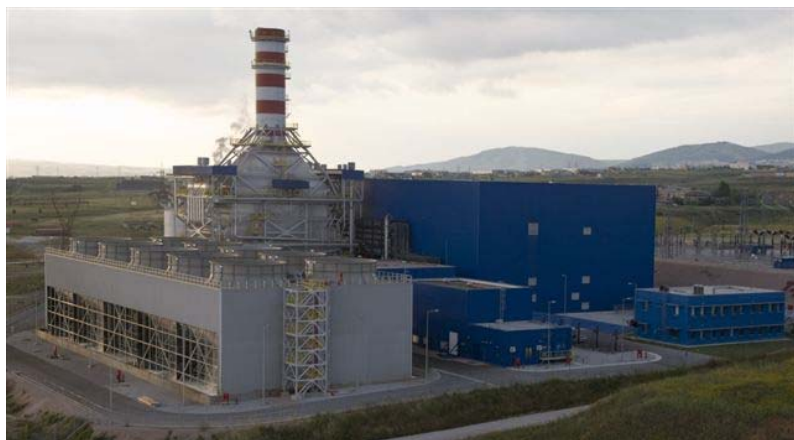
Thessaloniki 390MW CCGT power plant
